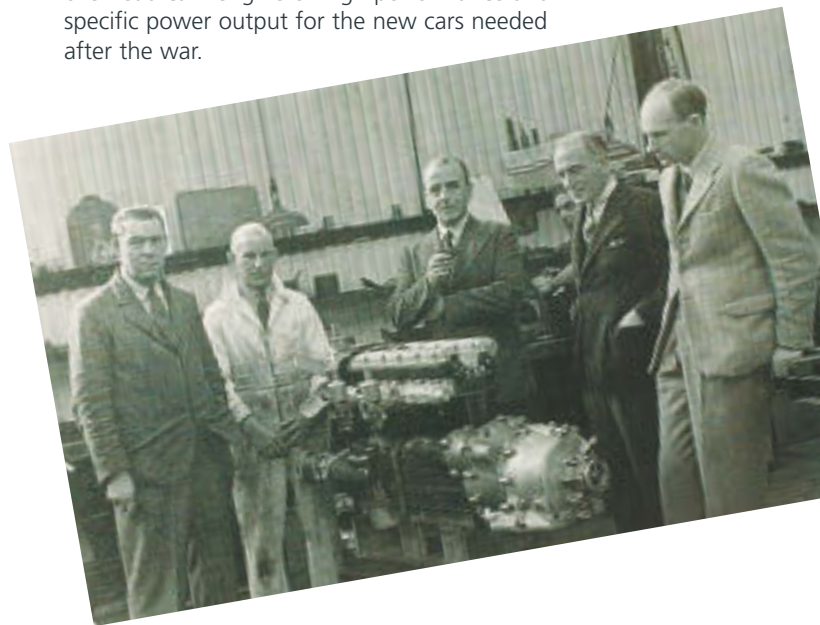
LB6 Twin Overhead Cam - Designed by WO Bentley it features a barrel crankcase design. Initially producing around 80bhp, it was to be developed in 3 litre form eventually to produce close to 230bhp in full racing trim
