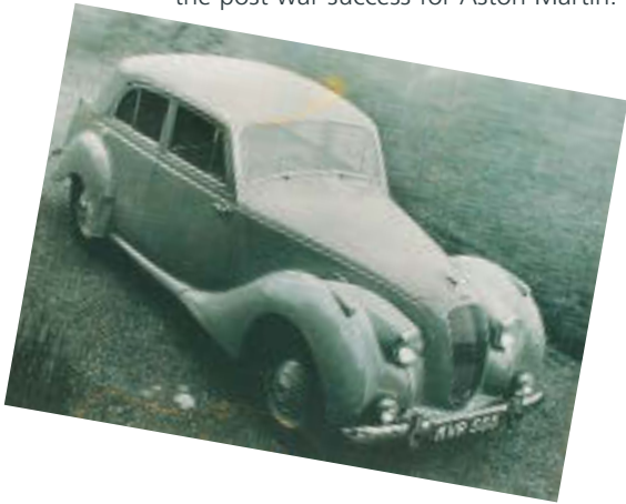
The first Lagonda to see production at the end of the 2nd World War. The chassis owed many of its design features to the LG6 pre-war Lagonda.
